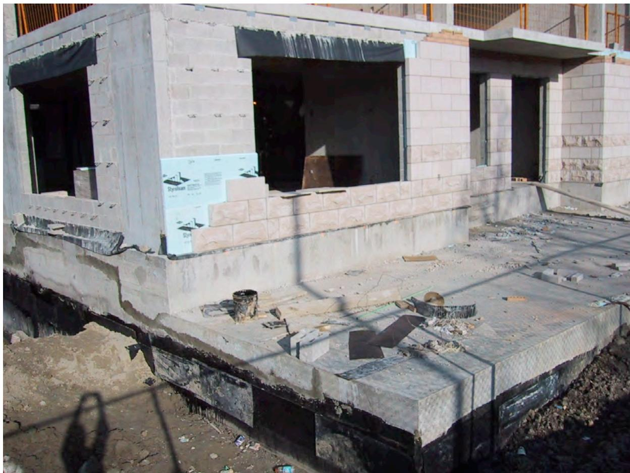
**Doing It Right** - Rare example of a condominium project where masonry block back-up is used behind the exterior insulation and brick facade. Note the use of punched windows instead of window wall assemblies from floor to ceiling. This type of construction provides superior durability and energy performance for a marginal premium.
